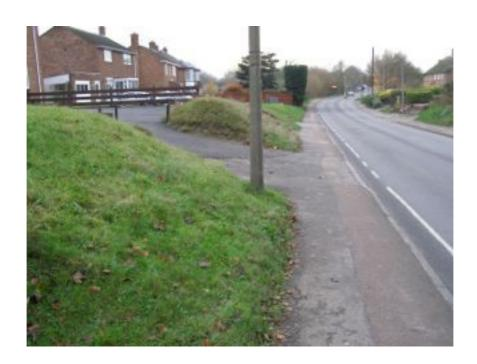
8 Cut back overgrown trees and widen path for cycle traffic. A conversation with a local resident suggests the boundary with local houses is at their fence, well back from the path.
